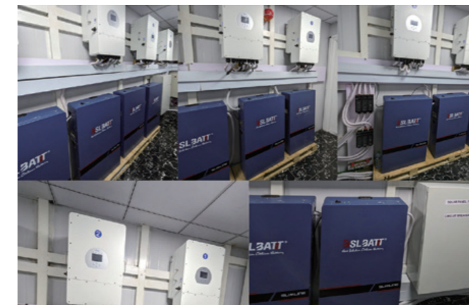
96kW Deye Inverter / 10*B-LFP48-300PW 153kWh / 120kWp Panel
